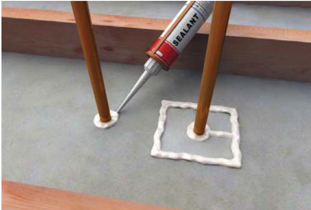
Figure 4 Sealing where pipes enter the roofspace
