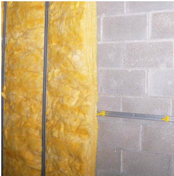
Figure 6 Internal dry-lining on blockwork with thermally efficient fixings
