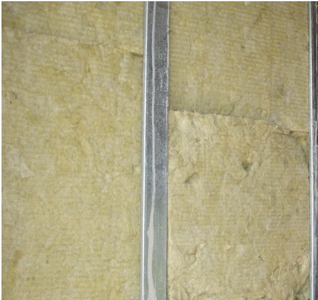
Figure 7 Tightly-fitting insulation in lightweight frame
