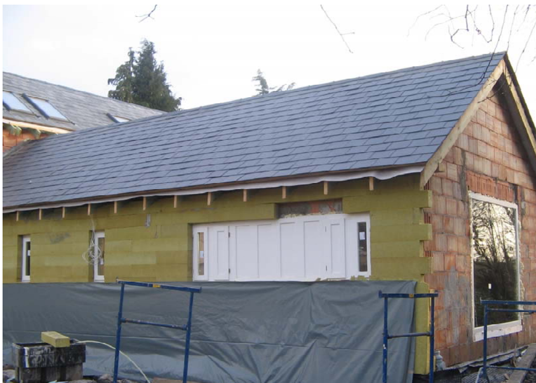
Figure 2 External insulation under installation
