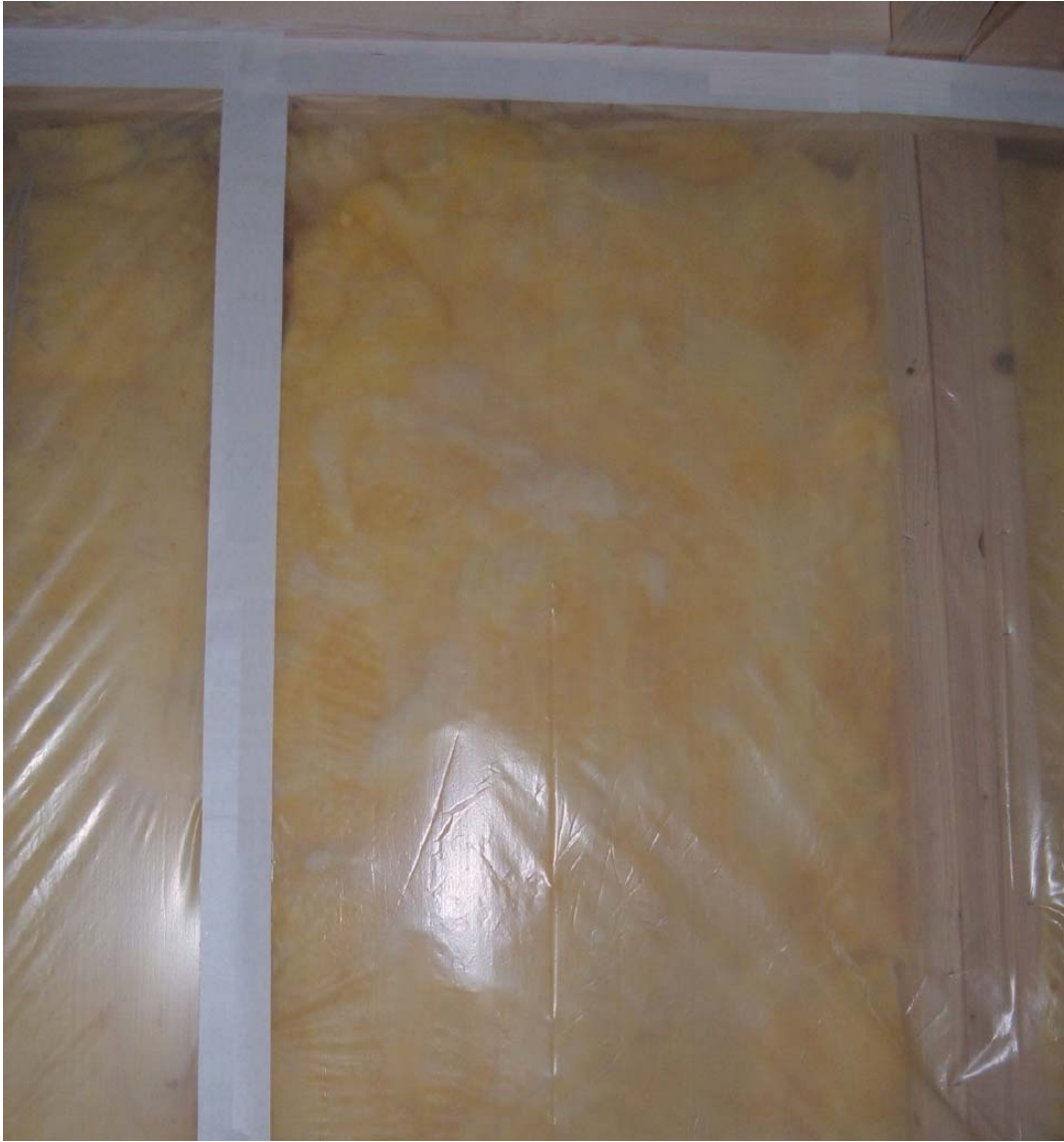
Figure 8 Joints sealed in air tight membrane
