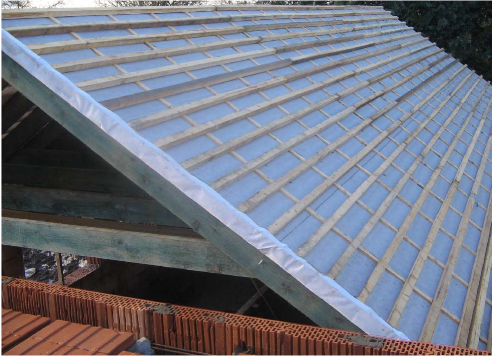
Figure 16 Roof with ventilated counterbattens and unventilated attic
