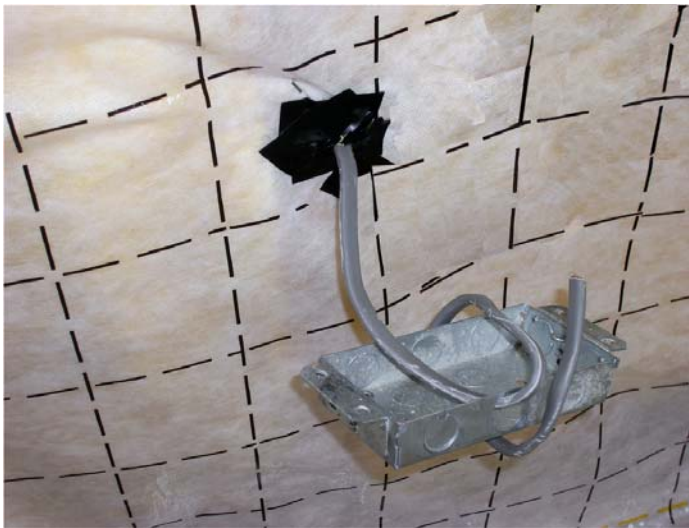
Figure 13 Sealing around connection to electrical socket outlet
